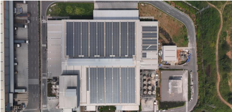
On-site solar - 38 mw capacity installed / under-installation
